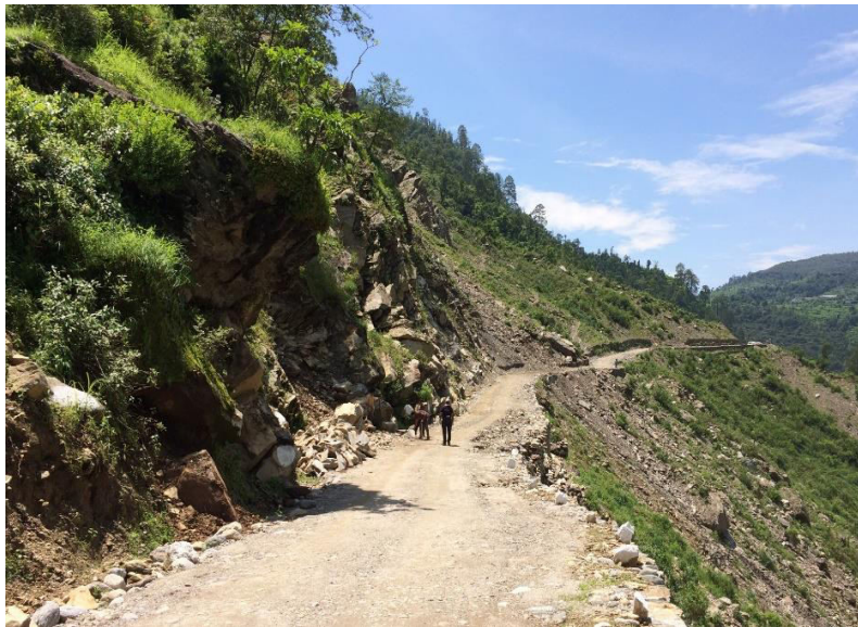
Figure.12 Another end of the slide zone with steep slope. Rocks are exposed along the road, followed by debris.
