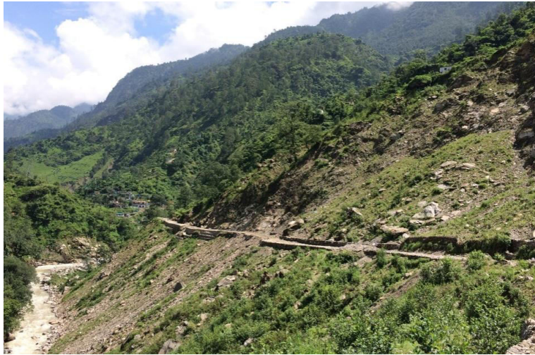
Figure.12 Another end of the slide zone with steep slope. Rocks are exposed along the road, followed by debris.
